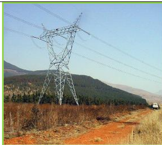
Figure 6: Photographic illustration of a Cross rope suspension tower.
